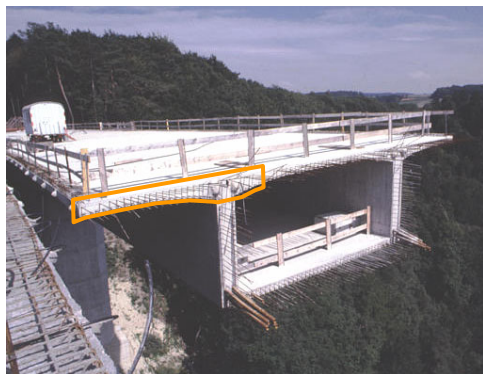
a) Bridge girder with cantilever
