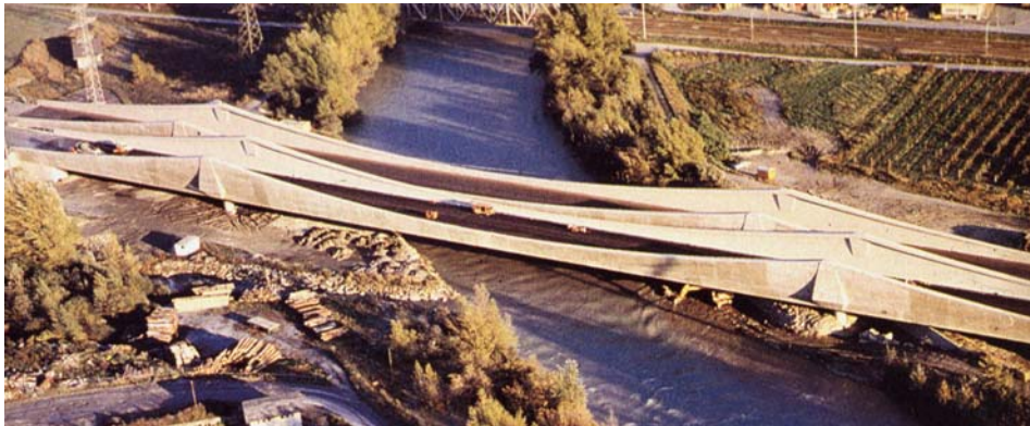
Figure 1: General view of the two Riddes bridges
