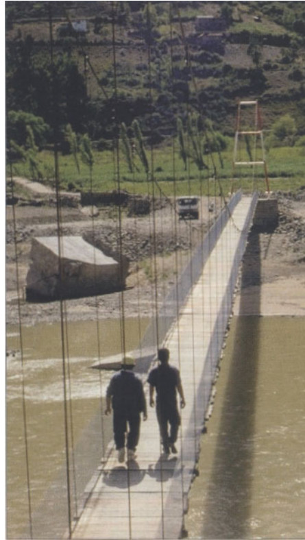
Fig. 3: The 100-m suspension bridge over the Rio Paute, Ecuador
