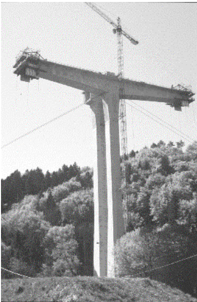
Fig. 7 Mentue bridges during the free cantilevering
