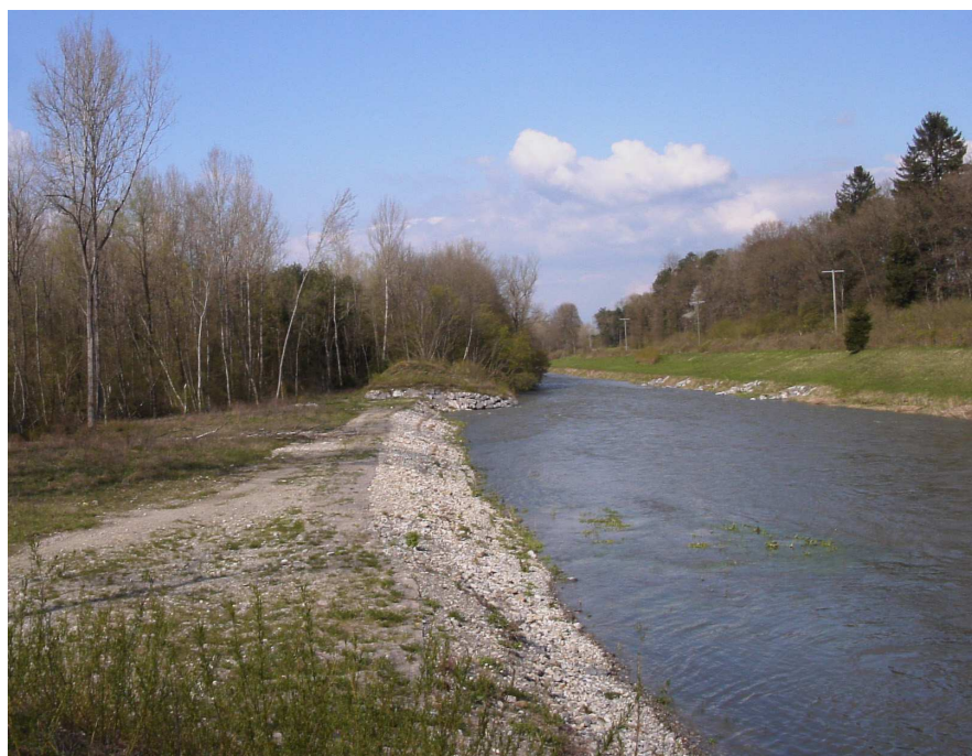
Figure 2.3: Overtopping dam on the river Broye, Payerne, Switzerland (photo: G. De Cesare).
