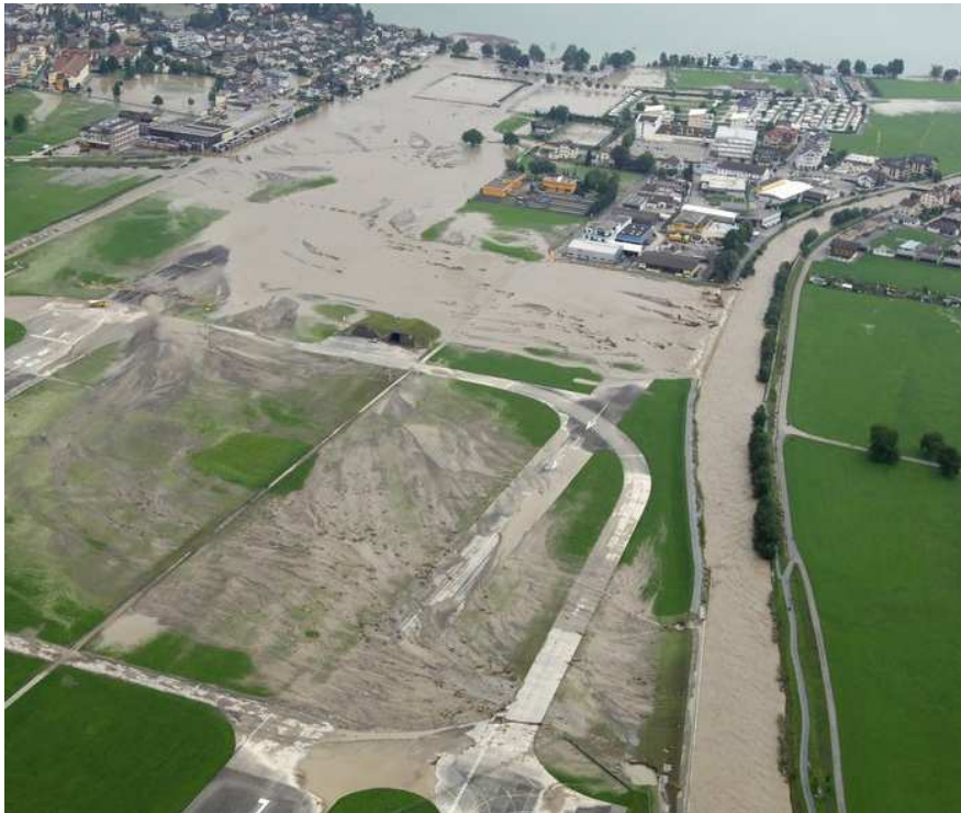
Figure 2.4: Side weirs equipped with tilting fuse gates on the river Engelbergeraa, centre of Switzerland (photo: Swiss air force).
