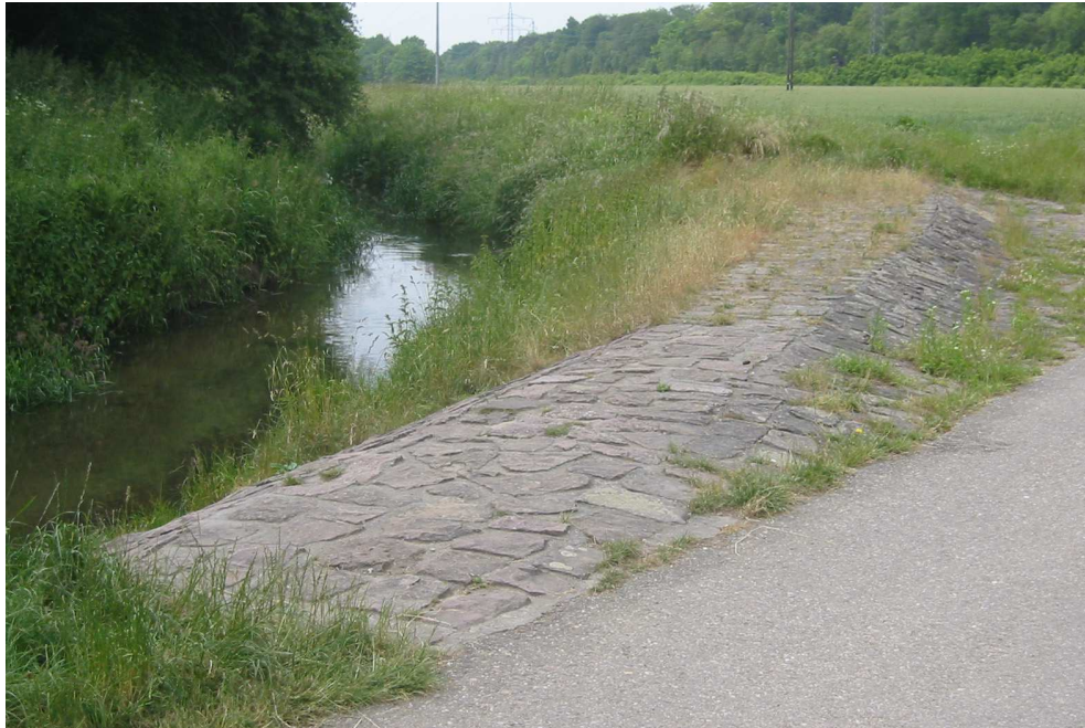
Figure 2.6: Side overflow dam on the river Erlengraben, Karlsruhe, south of Germany (photo: B. Rosier).
