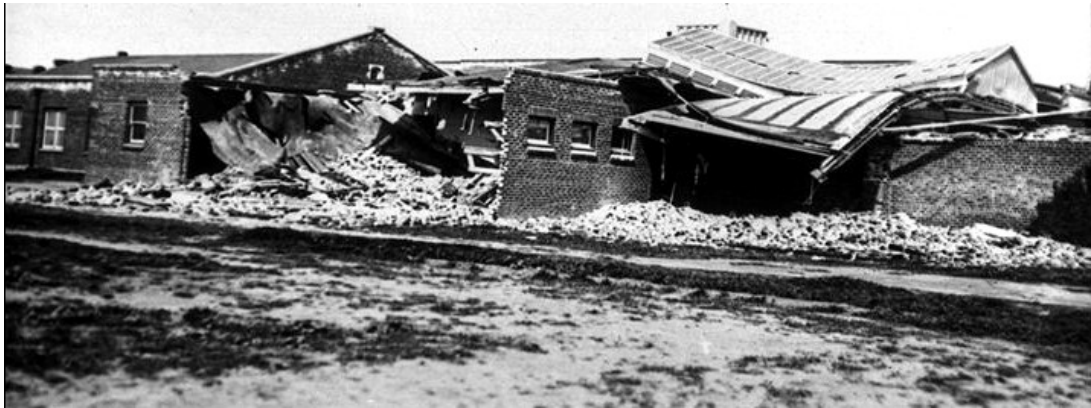
Compton Junior High School, Long Beach Earthquake, 1933
