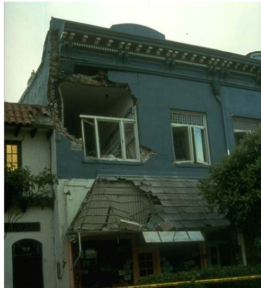
Santa Cruz Area, Loma Prieta Earthquake, 1989
