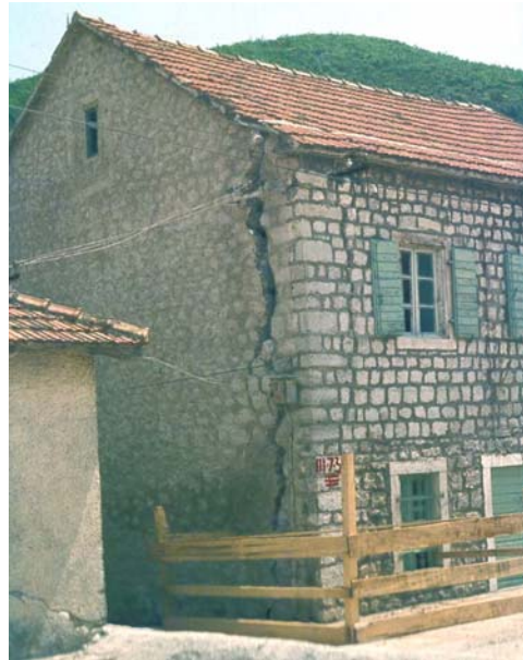
Figure 1.8: Montenegro, 1979: separation of walls at the corners (Courtesy of Tomazevic, personal communications)
