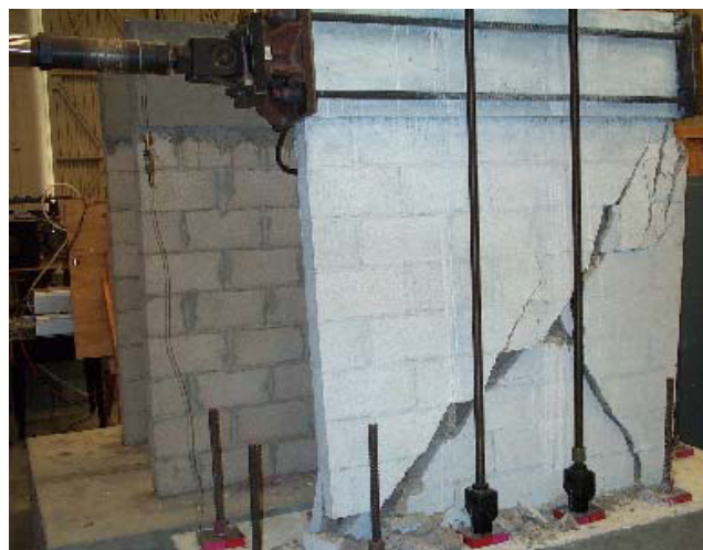
Figure 2.14: Shear failure of reference reinforced masonry wall [HMA 03]
