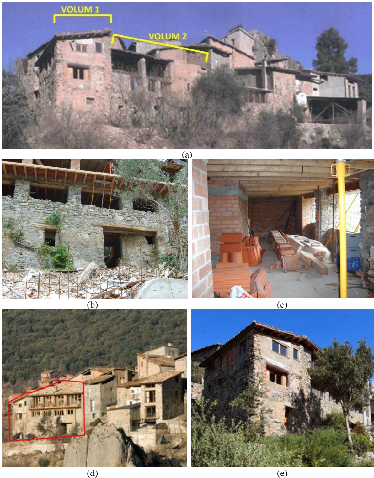
Figure 1: Images during the first renovation conducted in 2007 (a, b and c) and the current status (d and e).
