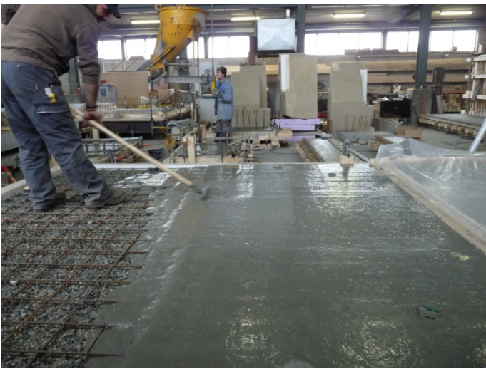
Figure 5. Placing of UHPFRC on large specimens
