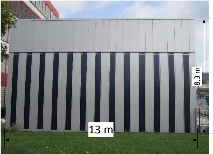
Figure 1: Cogeneration demonstration façade at Lucerne University of Applied Sciences. The TSC is placed in the upper part of the façade and supplies preheated outdoor air to the building. In the lower part, thin slice PV ribbons have been placed for solar power generation.
