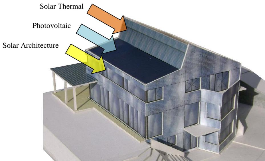
*Figure 1: Pilot and demonstration building (here a picture of its model) aiming at a 75% thermal solar fraction (heating and hot water), 25% are covered by wood pellets. The photovoltaic field covers the buildings electricity demand about four times. The construction will be/was terminated in summer 2013.*
