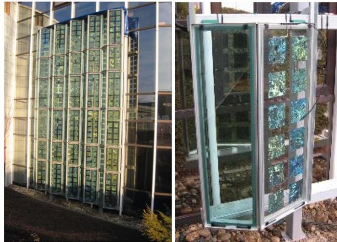
*Figure 2: Left: Prototype pleated double skin PV facade designed and constructed for the Ressources project. Right: single prism element showing PV and glazed surfaces.*
