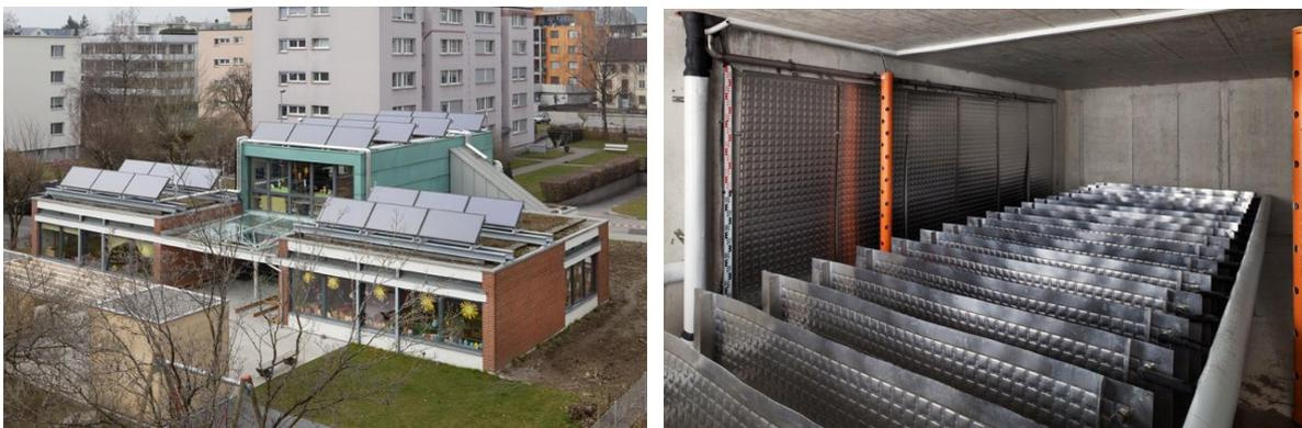
Figure 3: The collector field of the pilot plant on the roof of the kindergarten in Rapperswil SG (left) and view into the buried ice storage of the pilot plant before filling with heat exchangers at the bottom that can be iced and de-iced (right).
