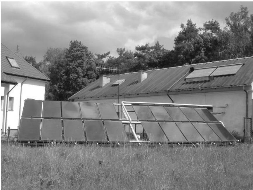
*Figure 1: The solar segments in the hybrid system.*
