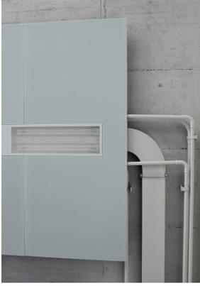
Figure 6: Photograph of radiant panels in HPZ building.
