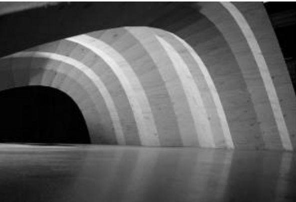
Figure 3 . Generated spatial structure made out of block timber panels
