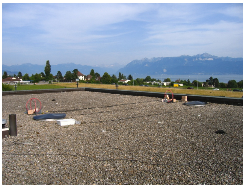
Fig. 6.2 Experimental setup 2 (a) and location of the sensors on the rooftop (b).
