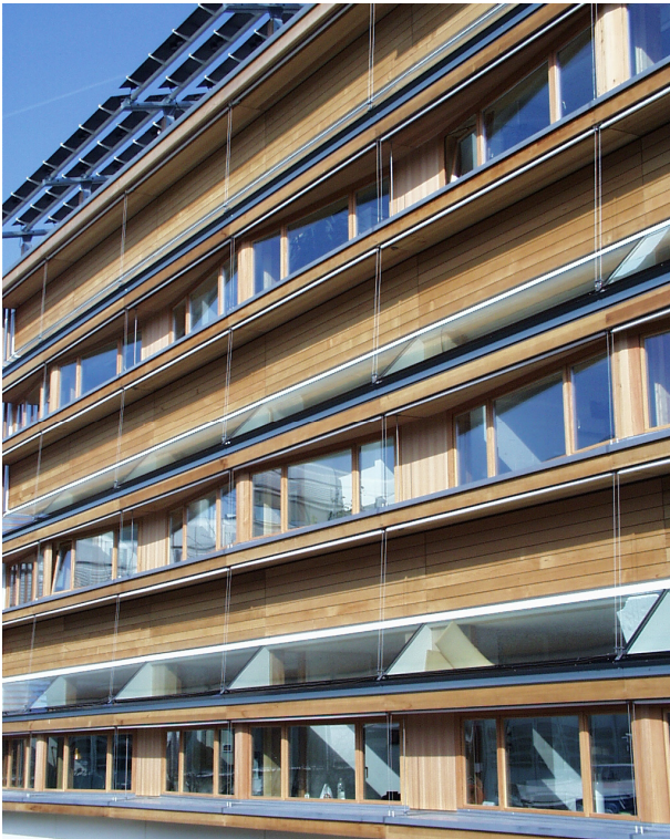
The anidolic daylighting façade of the LESO building
