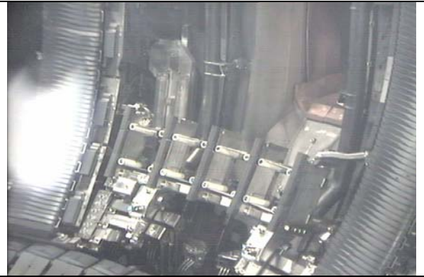
Figure 1. View of one group of four AE antennas as installed in vessel during June 2005.
