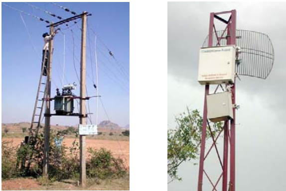
Figure 7a: AC Phase tap point. Fig7b: AC Neutral generated locally and connected to charger unit
