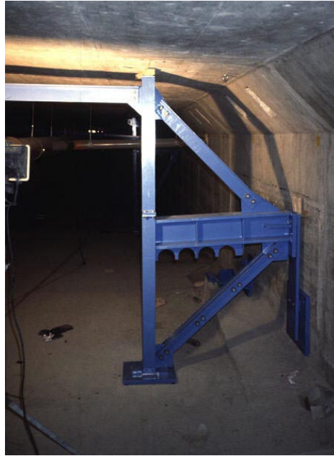
Figure 6: Vertical deviator for the parabolic post-tensioning
